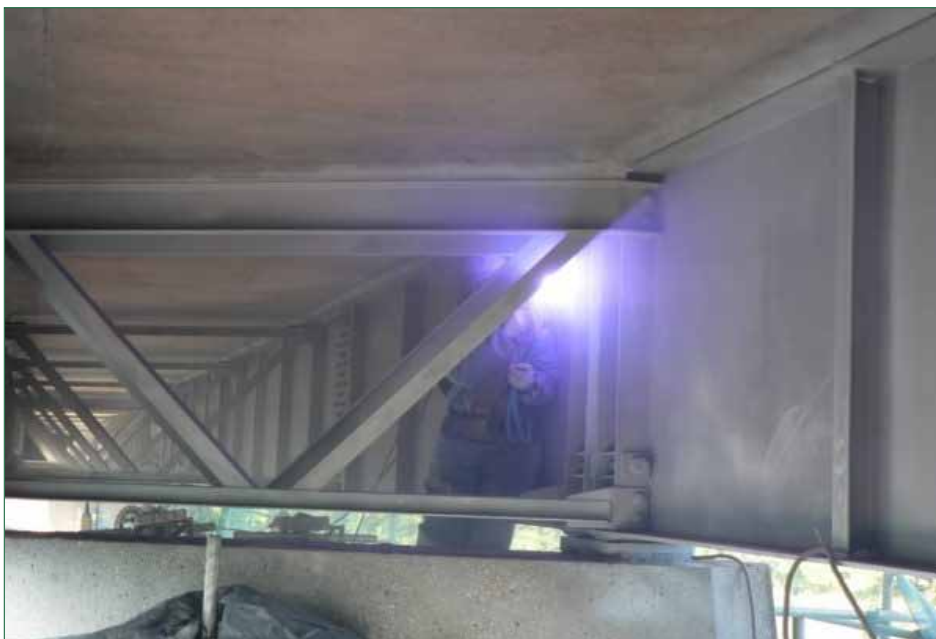
TMS being applied in situ to Puhoi Viaduct girder
