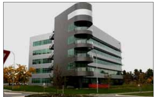
Aluminium alloy composite panel cladding on a modern building façade
