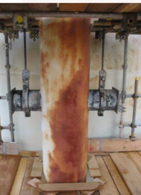
Figure 1 (referenced on page 71): pipeline corrosion in a natural gas liquids plant. Pipe and vessels repair prioritised over structural repairs.
