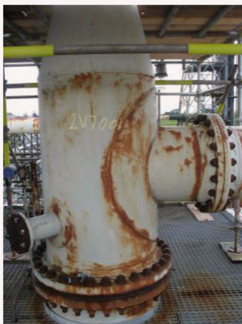
Figure 1 (referenced on page 71): pipeline corrosion in a natural gas liquids plant. Pipe and vessels repair prioritised over structural repairs.
