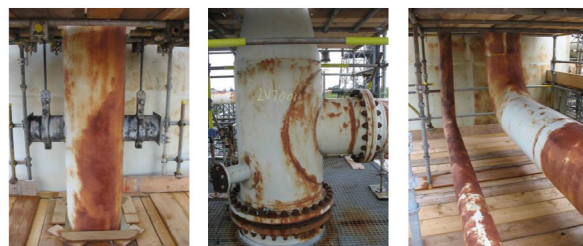
Figure 1: pipeline corrosion in a natural gas liquids plant. Pipe and vessels repair prioritised over structural repairs.
