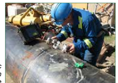
Non-intrusive ultrasonic measurement of corrosion occurring inside a pipeline
