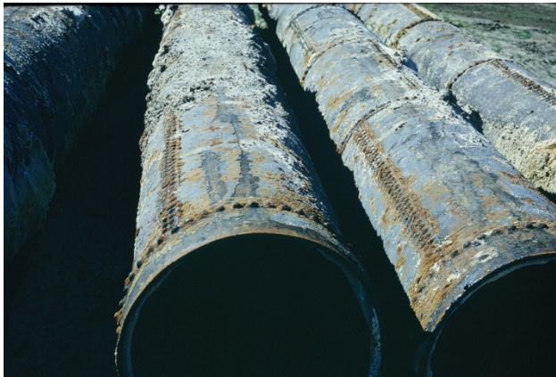
Figure A3 Riveted steel pipe
