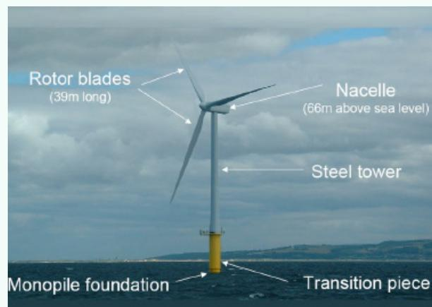
Figure 6: Components of a monopile offshore wind turbine
