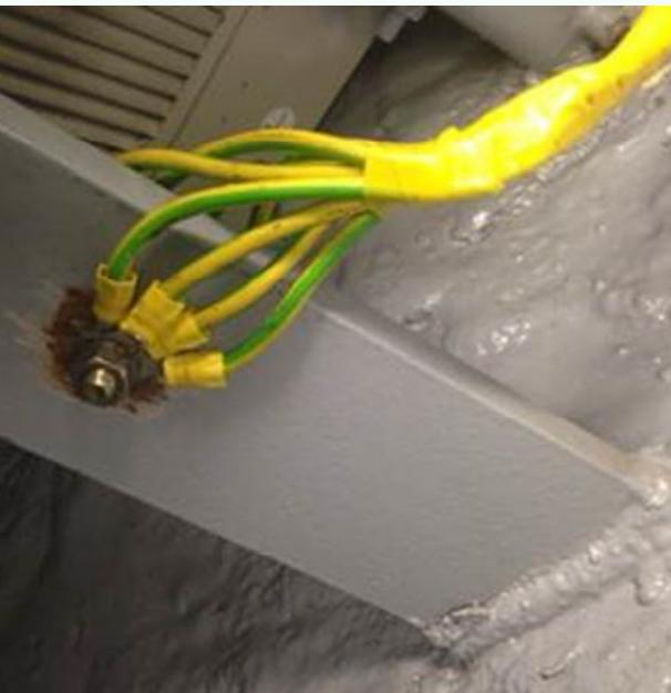
Figure 11: Earth cable termination point – note the small gauge wire and crimped connectors.
