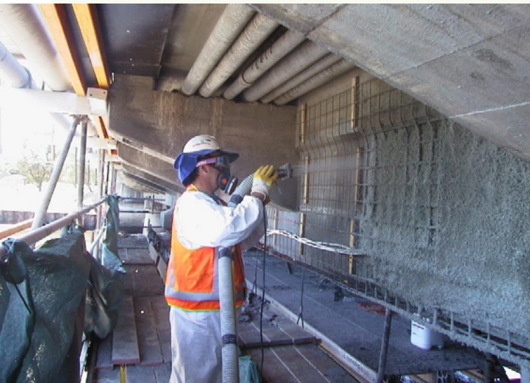
An Operator Applying Re-alkalisation to the Bridge (Photo circa 2001)
