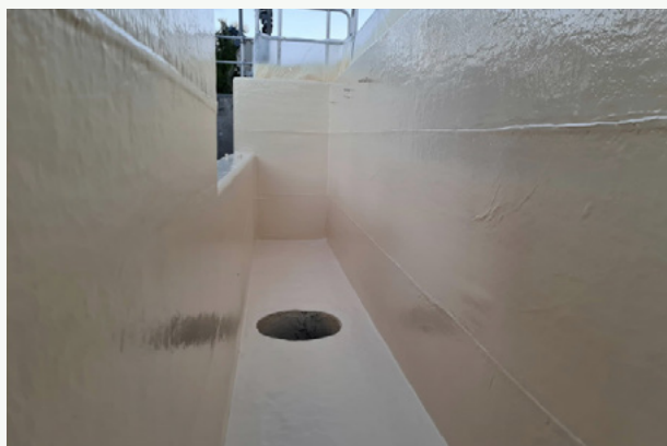
Completed Hybrid PU lining installed in inlet channel at Mackay South Water Recycling Facility.
