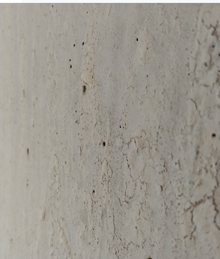
Figure 1: Dried residues of a Penkal Realkalization Solution application undertaken to a carbonated concrete wall prior to its washing off.
