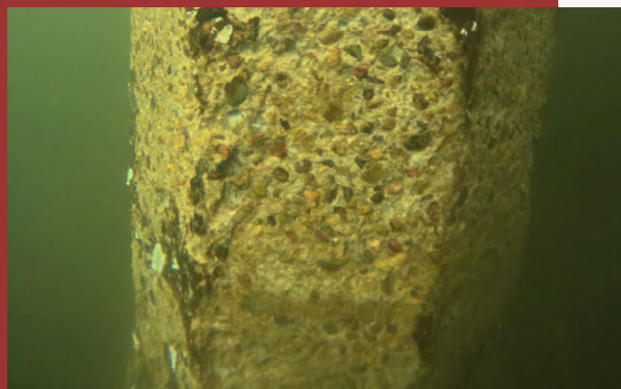
Figure 1 (top): Concrete deterioration on underwater piles.
