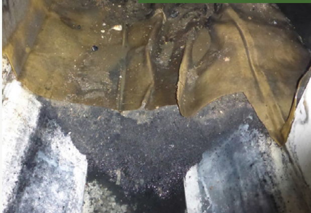
Failed Pure Polyurea linings at Mackay North Water Recycling Facility.
