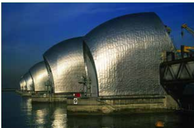
316 stainless steel cladding on Thames Barrier
