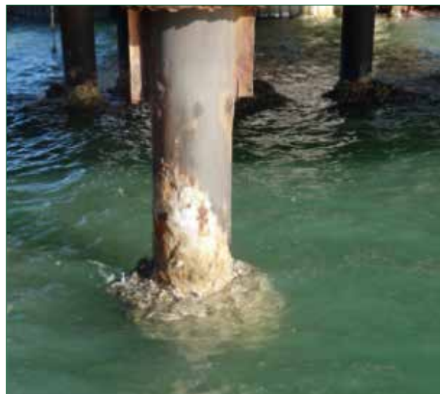
Heavy layer of calcareous deposit and substantial marine growth on a wharf pile. (from the paper by Bruce Ackland on the ACA website. Weblink above).
