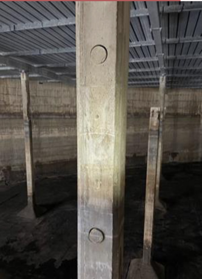
Figure 3 Example of cores taken locations below the water line and above the water line
