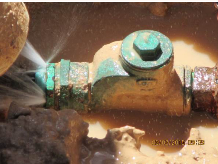
Figure 3: Leakage of PE main-to-meter connection at ferrule.
