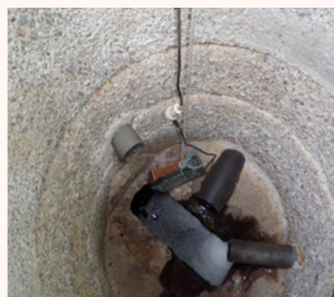
Fig 2. Corroded manhole
