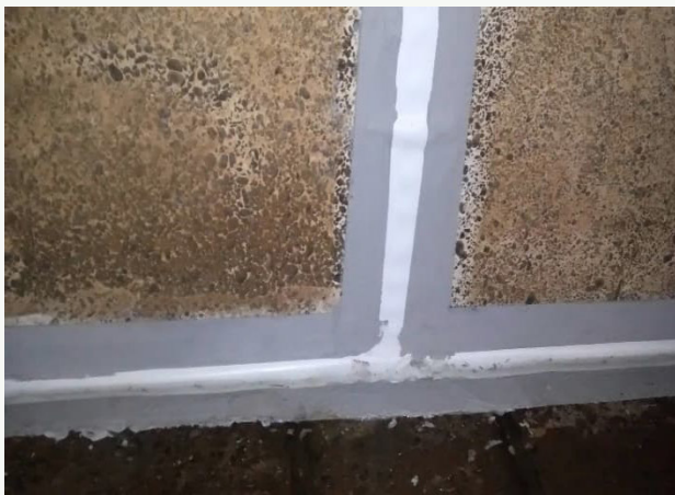
Hypalon Bandage system (bonded using epoxy paste) installed to vertical joints and wall/floor intersection.
