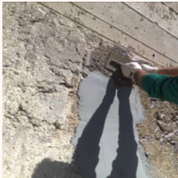
Fig. 1 Repair of Abrasion Damage on inclined Screw Pump trough
