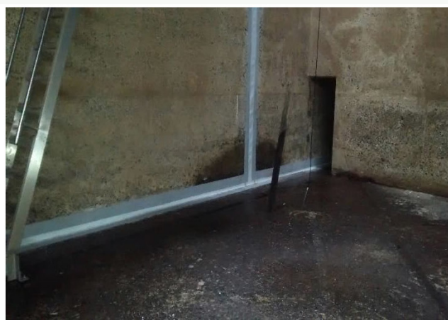
Hypalon Bandage system (bonded using epoxy paste) installed to vertical joints and wall/floor intersection.
