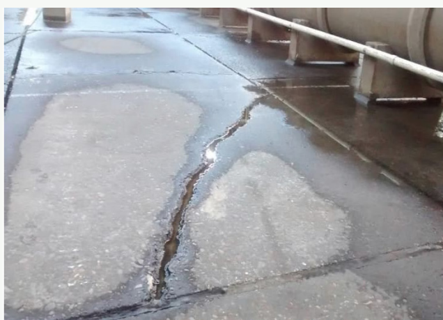
Cracks in existing concrete floor slabs
