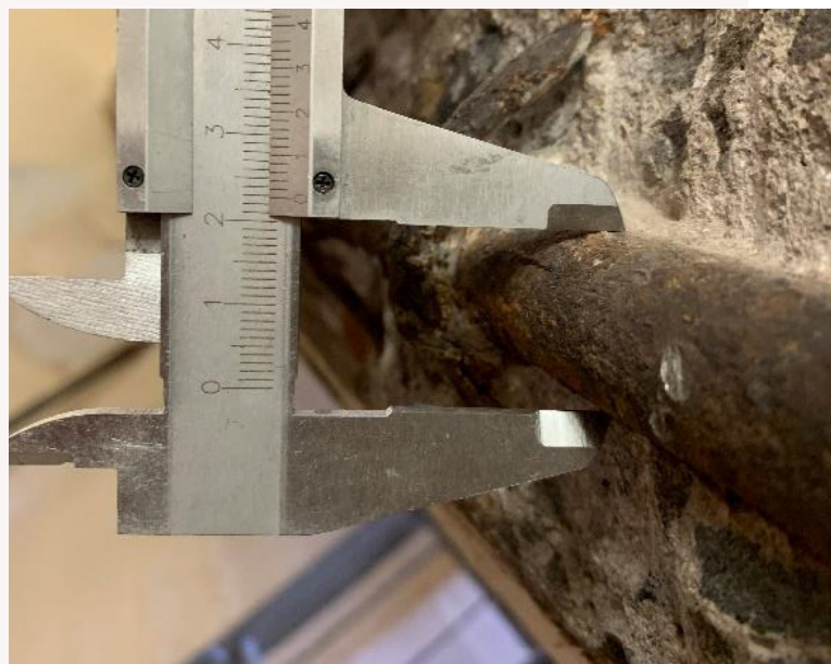
Figure 5 - Inspection Of Rebar At Areas Of Spalling
