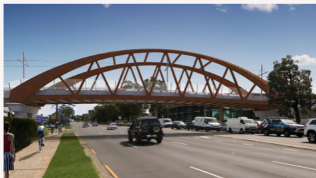
JAMES RUSE DRIVE LIGHT RAIL BRIDGE, PARRAMATTA, NSW (2021)
