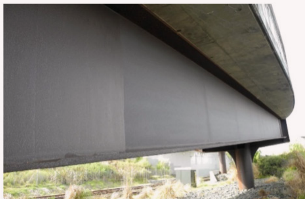
MERCER RAIL OVERBRIDGE, SOUTH OF AUCKLAND, NZ (2006)
