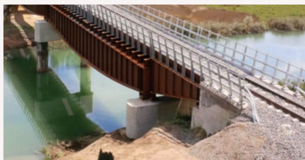
NZ RAIL REPLACEMENT BRIDGE (2012)
