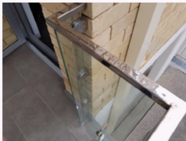
Figure 13: Contrast high sulphur (left) and low sulphur (right) with similar washing after one year but no prior pickling
