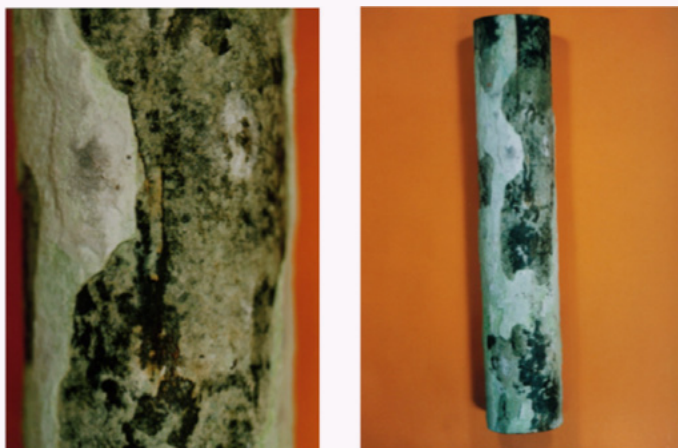
Figure 2 A & B: Pipe with only longitudinal cracks and layered scale
