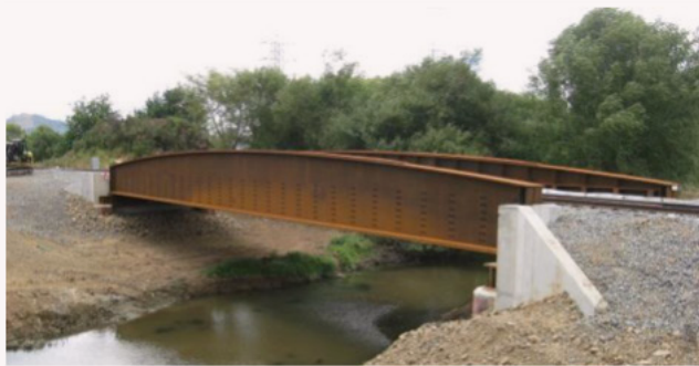
NZ RAIL REPLACEMENT BRIDGE (2012)
