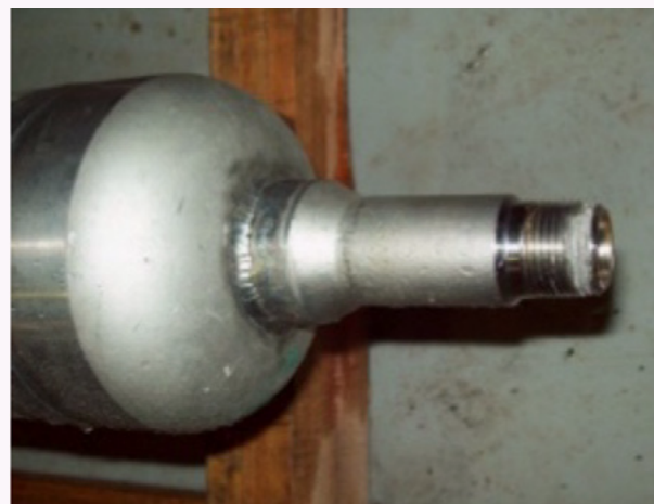
Fig 9: PTFE tape sealing (and corroding) 2507 Super duplex in seawater
