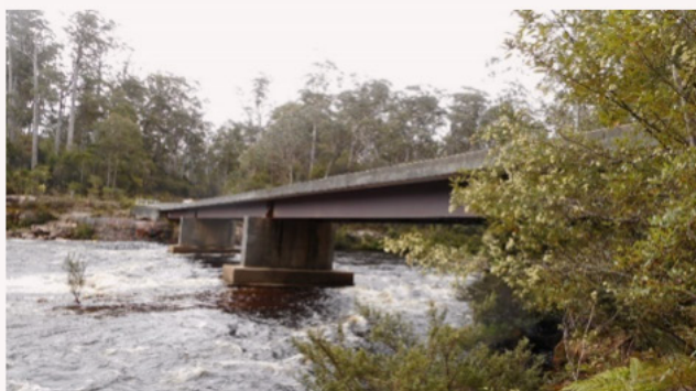
PICTON RIVER BRIDGE, TASMANIA (1981)
