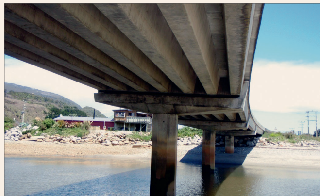
Underside of the Ngakawau River Bridge showing the good condition of the U-beams.
