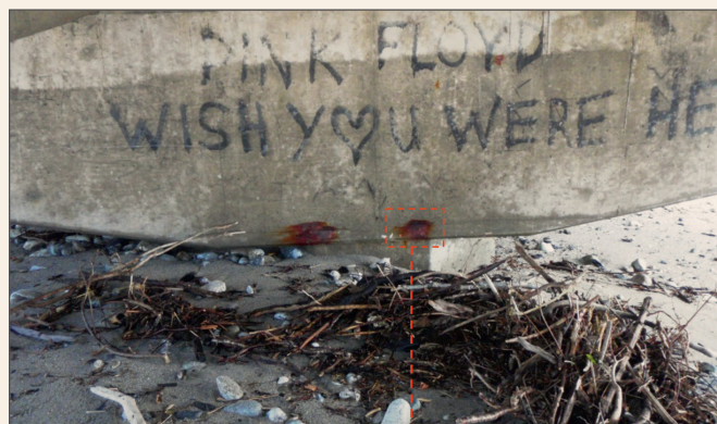
Underside of the Ngakawau River Bridge showing the good condition of the U-beams.
