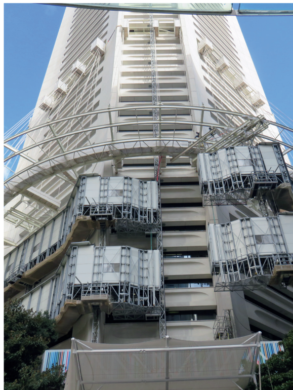
Front Cover Photo: MLC Façade Maintenance Project - Transfer of Mast Climber Work Platform via Suspended Monorail System. Photo: D. Lambert.
