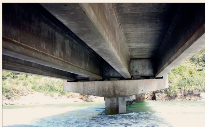
View of the underside of Fox River Bridge showing the simply-supported pre-stressed I-beams.
