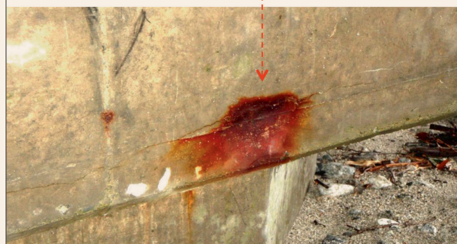
Spalling at base of the hammerhead on Pier C on the Fox River Bridge.
