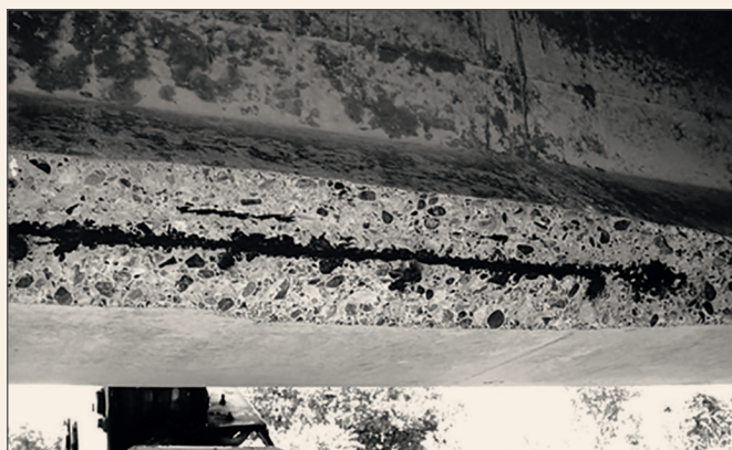
Underside of the Ngakawau River Bridge showing the good condition of the U-beams.
