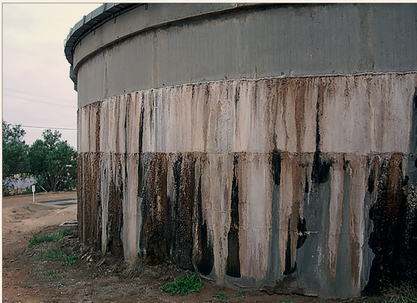
Figure 9. 'Black rust' (magnetite) localised corrosion of steel reinforcement due to leaching at construction joints in the wall of a reinforced concrete tank containing potable water. (Photo courtesy of Greg Moore)
