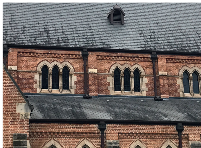
St George's Anglican cathedral was reroofed in original Welsh slate eight years ago. During a rare rain event the beginnings of bacterial attack are showing other than the run-off from copper dormers which have a biocidal impact on the microflora Courtesy Ian MacLeod.
