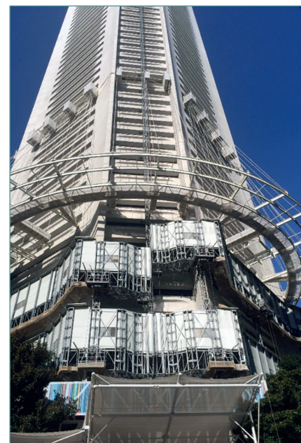
Figure 3 – Monorail Transfer of platforms between phase 1 and 2 of the project.
