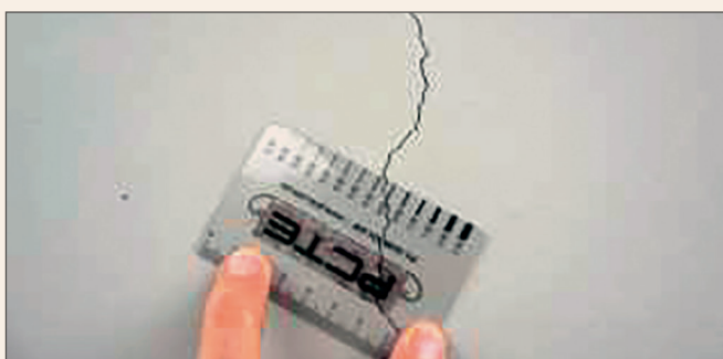
Crack (0.40 mm) on north face of pier wall.
