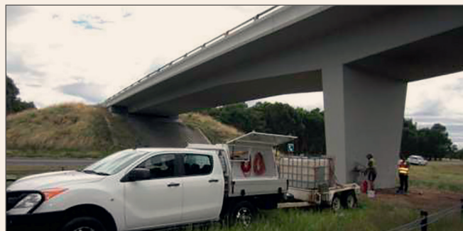
Bridge viewed from west and core drilling on the south side of the pier wall.
