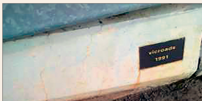
Crack (0.35 mm) on south face of pier wall.
