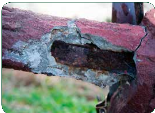
Decorative concrete fence undergoing significant corrosion at seaside resort
