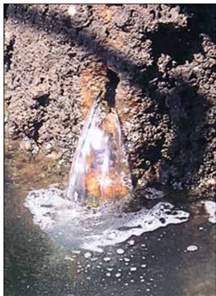
Example of ALWC with ground water running back into Newcastle harbour at very low tide.
