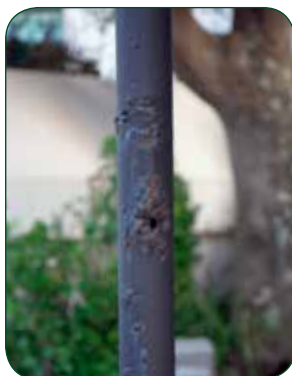
Corroded lamp post at seaside resort
