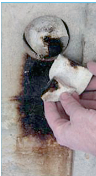
Corrosion stains of Oamaru Stone at the Hunters Building, Victoria University.
