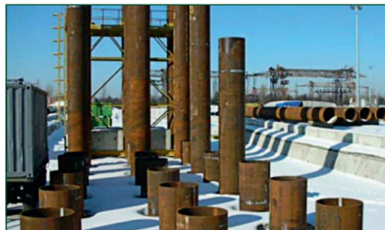
400 x 1m Piles Driven 26m into the Ground.
