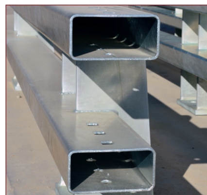
Figure. With a specified minimum HDG coating thickness of 85µm, AS/NZS 2312.2 can be used to estimate this bridge rail will be protected from rust for over 50 years in a C3 (medium) environment.
