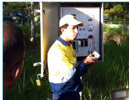
Nick Doblo explaining what potentials are used to protect a pipeline through a Transformer Rectifier.
