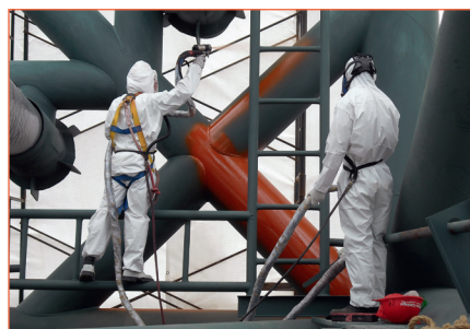
Corrosion protection on an oil & gas platform.
