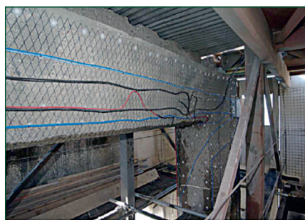
Figure 5 - Coated Titanium Mesh Anode Application.
