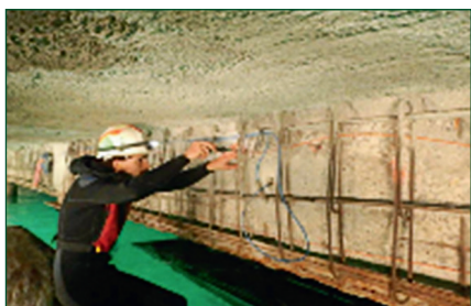
Conductor Installation.
