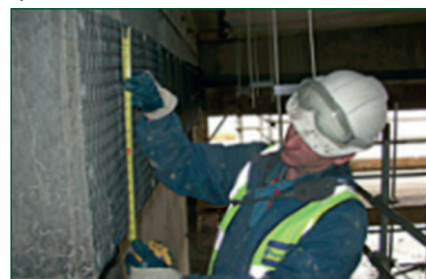
System Anode Mesh Installation.
