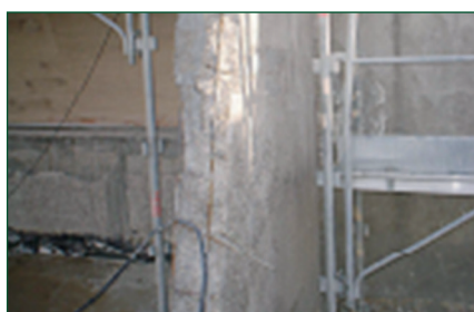
Defective Concrete Removed & Remediated.
