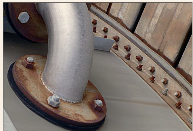
Figure 8 Dissimilar metal corrosion of a mild steel flange plate that is welded to a stainless steel pipe. Pipe appears to be insulated from the tank.
