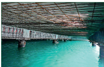
Concrete Removal and Rebar Replacement.
