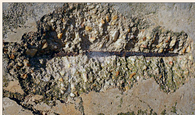
Figure 3 Reinforcement corrosion resulting in spalling concrete on external tank wall.
