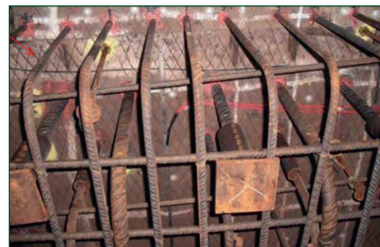
Titanium mesh based anode to be installed at the interface of concrete substrate and new corbels.
