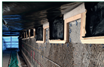
Mesh Overlay CP System.
