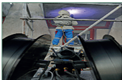
Thermal Spray Applied Zinc CP System.
