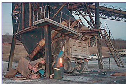
Figure 1. Collapse of steel salt bin in US that killed a truck driver. The road salt bin structure failed due to corrosion.
