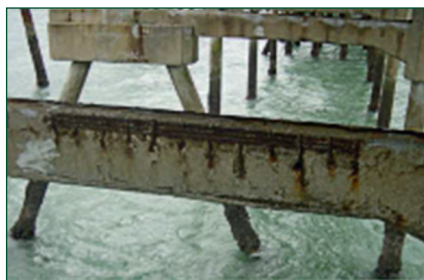
Corroded Rebar & Degraded Concrete.
