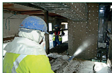
Sprayed Concrete Application.
