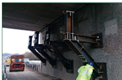
Temporary Support & Jacking Placement.
