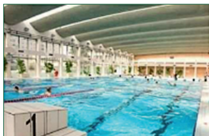
Prefabricated Prestressed Concrete Shell Roof Construction.
