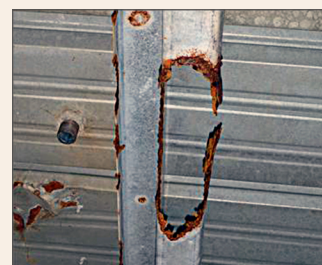
Figure 11 Corrosion of tank roof purlin, a galvanized Z-section, with complete section loss.
