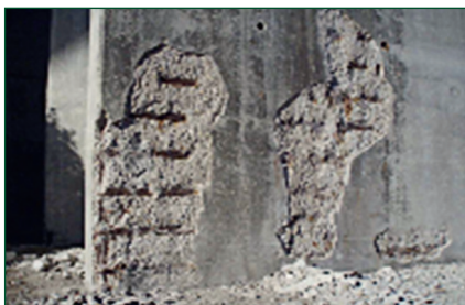
Corroded and Degraded Reinforcement.
