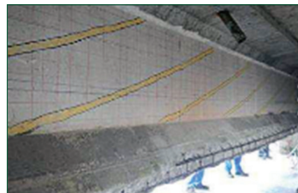
Post Tensioning Locations Marked.
