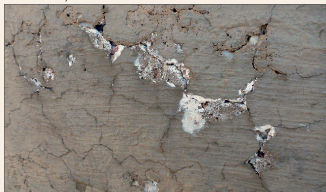
Figure 6 Suspected AAR cracking of concrete water tank constructed from locally sourced aggregate.
