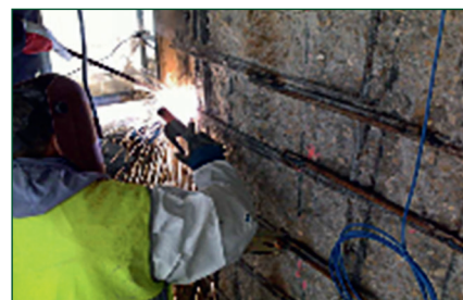
Anode & Reference Electrode Installation.
