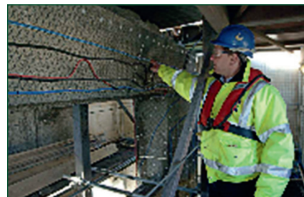
Titanium Mesh Installation.
