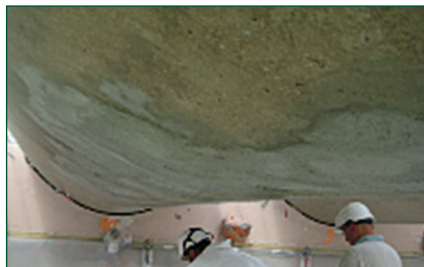
Concrete Patch Repair.
