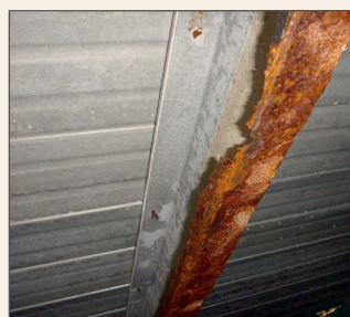
Figure 10 Corrosion of tank roof purlin, a galvanized C-section.
