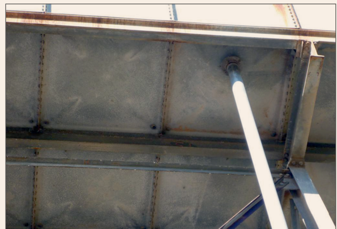
Figure 7 Atmospheric corrosion of galvanized coating, accelerated by the micro-environment on the underside of the tank (condensation, sun exposure etc.).
