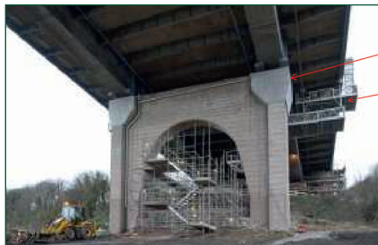
Corbel addition within clearance of the inspection gantry.
