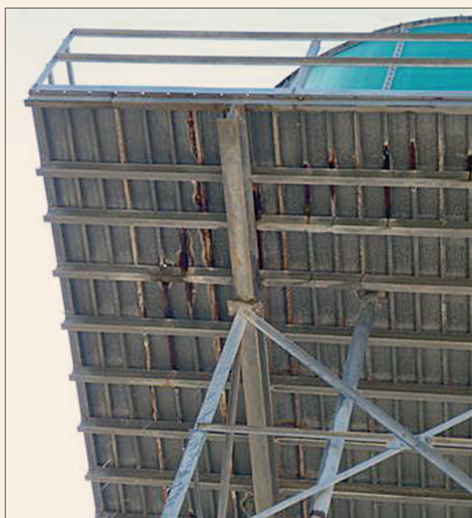
Figure 12 Corrosion of tank stand platform sheeting.
