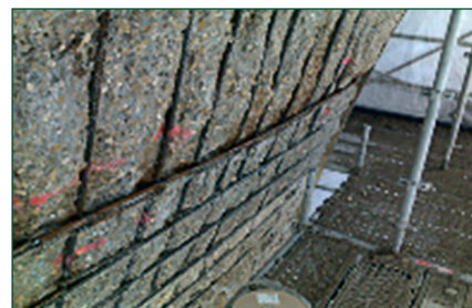
Hydro Demolition and Rebar Replacement.
