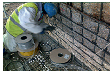
Titanium Ribbon & Anode System Placement.
