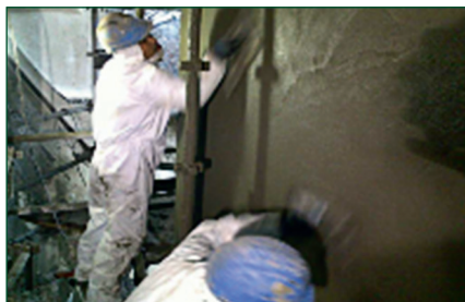
Trowel Finishing of Shotcrete.
