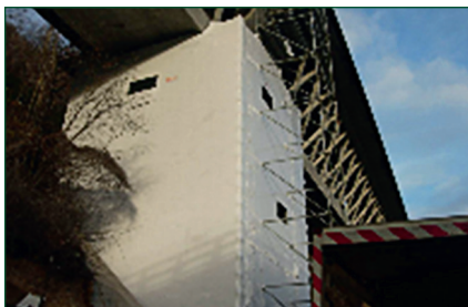
Sheeted and Heated Scaffold.
