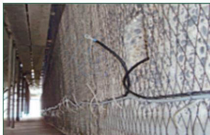
Installation of Impressed Current CP System
