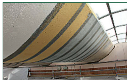
Applied Waterproof Membrane.
