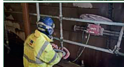
Titanium ribbon based anodes to be installed within slots cut into the concrete cover.
