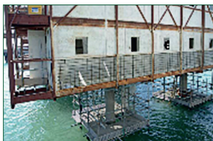
Encapsulation of Headstocks.
