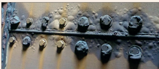
Figure 9 Blistering of internal coating at plate edges / bolt holes following immersion service.
