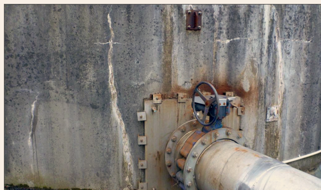
Figure 4 Cracking caused by early age thermal restraint in a reinforced concrete tank.
