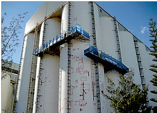
Figure 7 – 'Prototype' phase profiled mast climber system.
