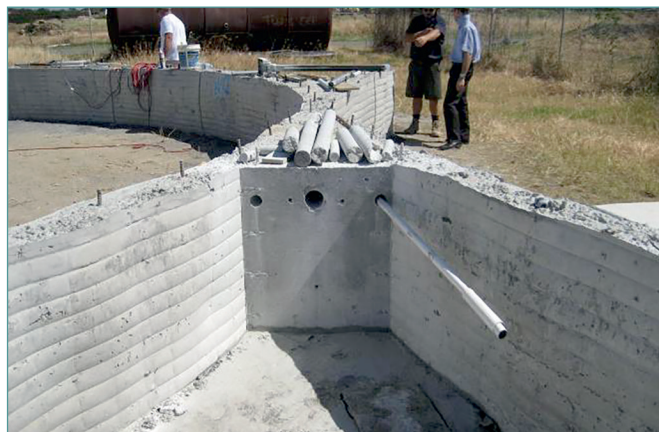
Figure 2 – Cored tendon placement holes.
