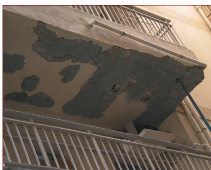
Soffits severely corroded due to roof leakage into a residential building.
