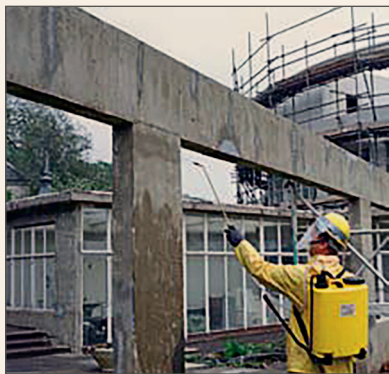
Figure 6: 'Topical' application of migrating organic inhibitor to concrete.
