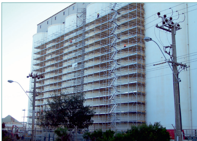
Figure 9 – Typical scaffold access on site (prior to encapsulation).
