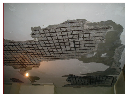
Soffits severely corroded due to roof leakage into a residential building.
