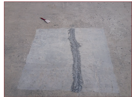
Surface grinding to open the face of the crack and sealing with epoxy resin.
