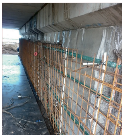
Cathodic protection to bridge piers affected by cracks, corrosion and spalled concrete, using embedded galvanic anode units (top) and distributed galvanic anode system (bottom).
