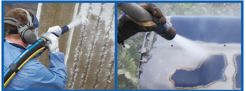
Concrete Surface Preparation
