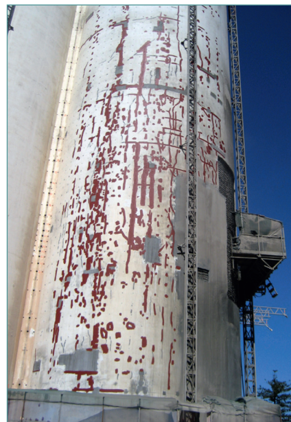
Figure 5 – After Kevlar tape removal from side of Silo 7.8.
