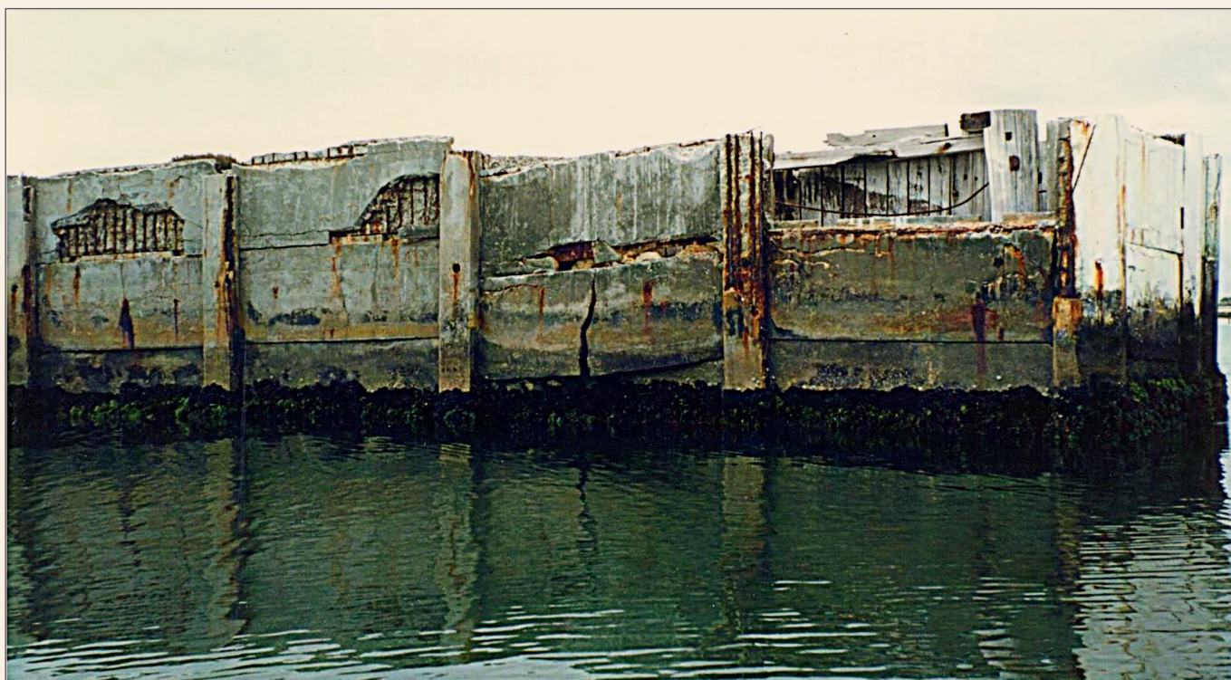
Figure 1: Reinforcement corrosion induced deterioration.
