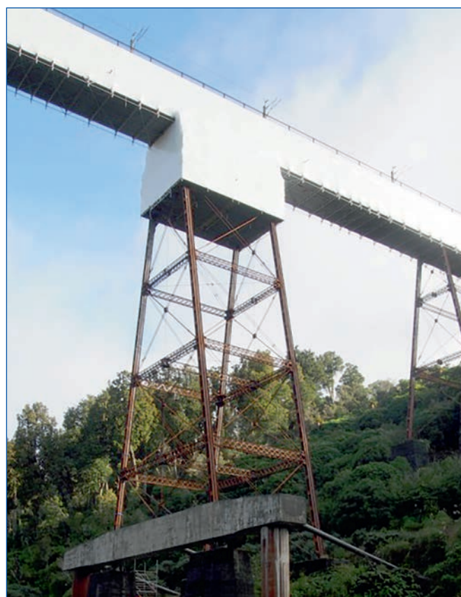
Figure 15: Encapsulation around Pier 7.
