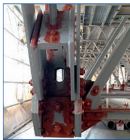
Figure 13: Tie Bracket and bottom chord washer plate.
