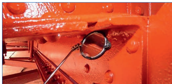
Figure 11: Inspecting Rivets for Paint Film.
