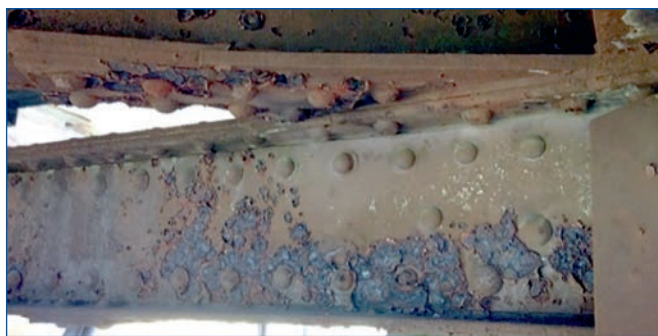
Figure 3: Heavy corrosion
