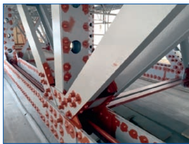
Figure 12: Strut and bottom chord strengthening.
