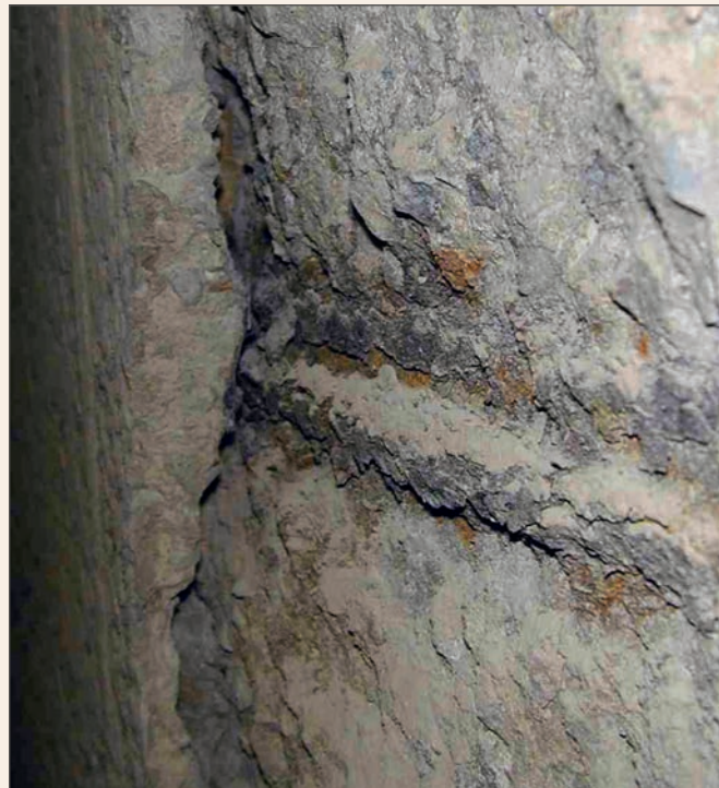
Figure 2. Carbonation induced spalling.
