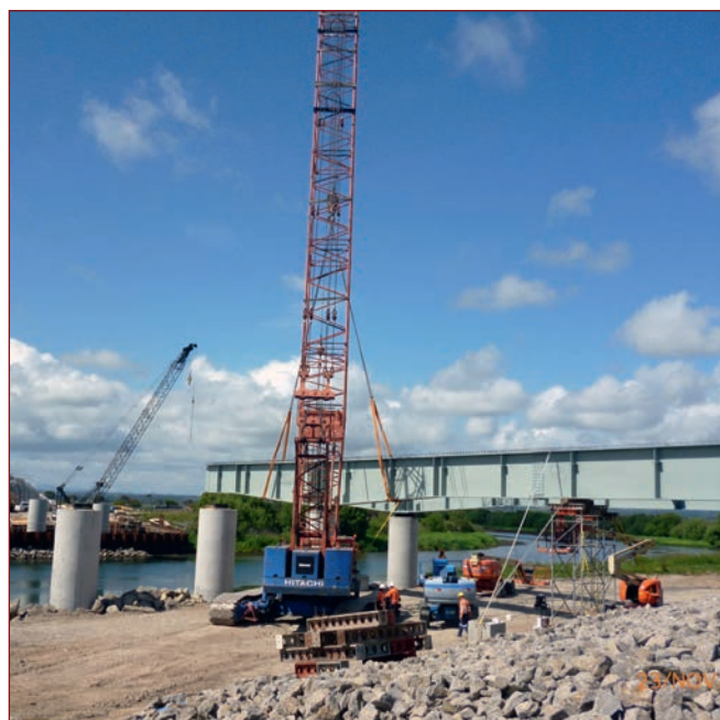
NZ Bridge over the Kaitung River coated with IZS in 2012.
