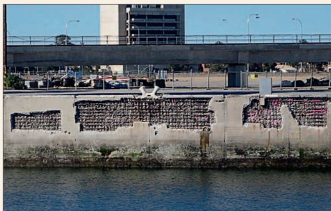
Figure 1. Result of chloride attack on a wharf structure,
