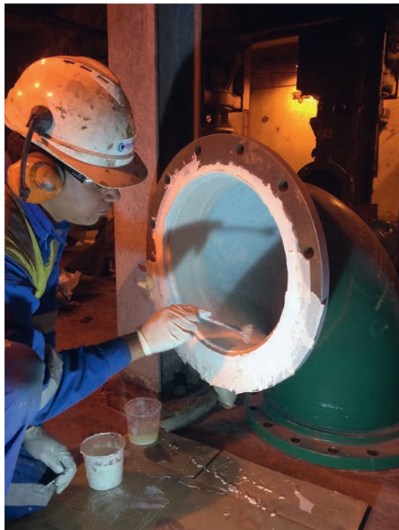
Front Cover Photo: In-situ field fit flange and rebate internal coating repairs using Chem-tect RB300 Photo by Greg Bladowski/Chemco.
