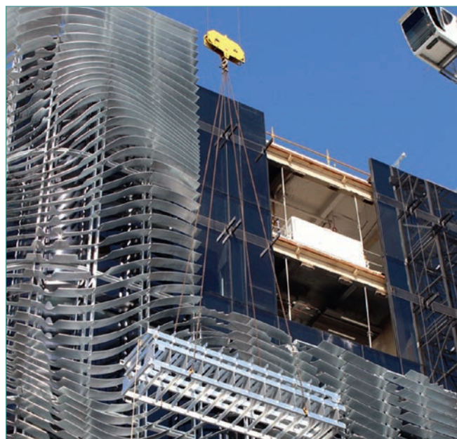
Sections of the galvanized façade being lifted into place by crane.
