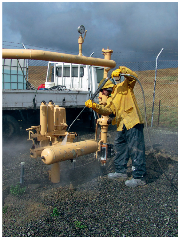
Front Cover Photo: Low pressure water washing a natural gas main line valve, after an algacide application. Photo courtesy Craig Ross at NSB Infrastructure.
