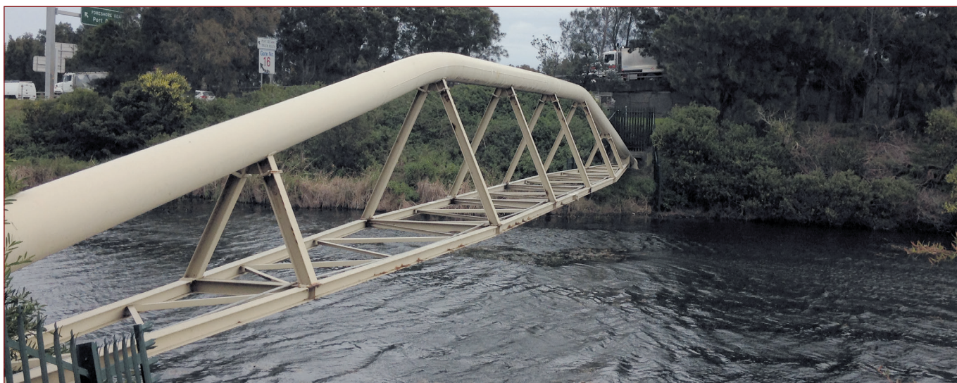
Pipe bridge crossing body of water.
