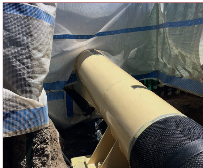
The above ground pipe section recoated.
