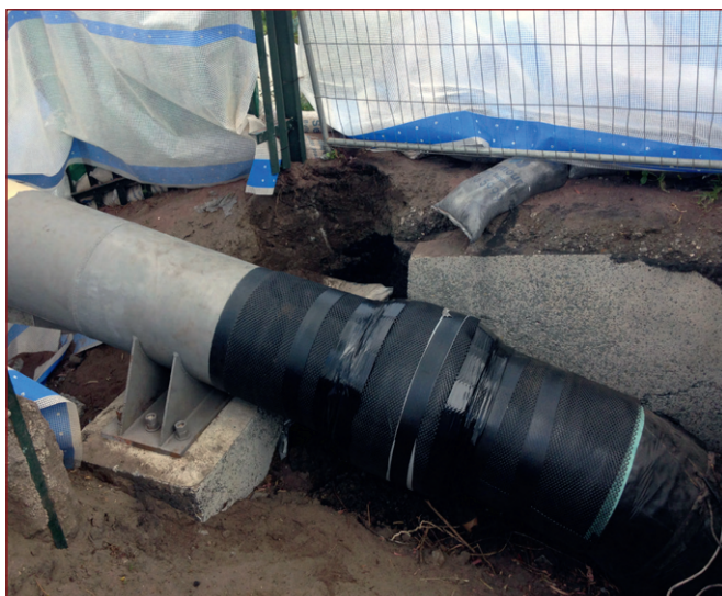
Pipe cleaned and recoated.
