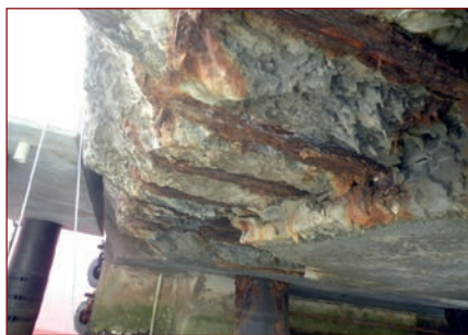
Figure 17. Delaminated concrete with heavily corroded reinforcing bars exposed.
