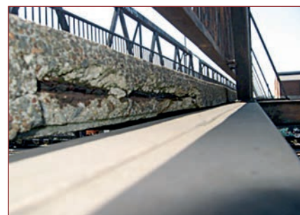
Figure 12. Walkway slab edge spalling and delamination.
