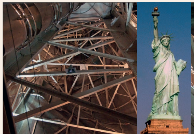
The 1986 restoration of the Statue of Liberty used duplex stainless steel to replace much of the original iron ore support framing. Photos © Mike Renlund and Erik Cleves Kristensen (inset).
