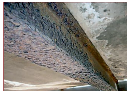
Figure 11 Heavy corrosion to walkway slab support beams.
