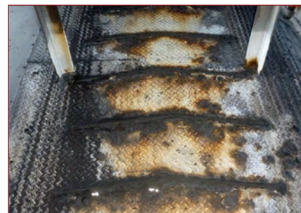
Figure 4. Corrosion to walkway floor plate, namely the heat affected zones, leading to perforations.
