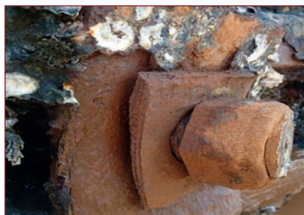
Figure 14. Corroded land tie fastener.
