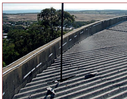
Figure 7. Failed vertical stressing bar of a 50ML reservoir located in the central coastal area of Queensland.
