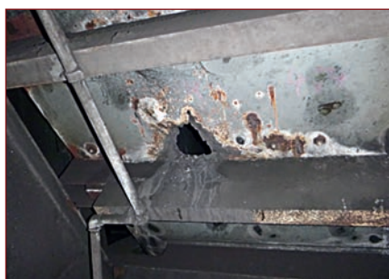
Figure 5. Heavily corroded and perforated bin wall plate element.
