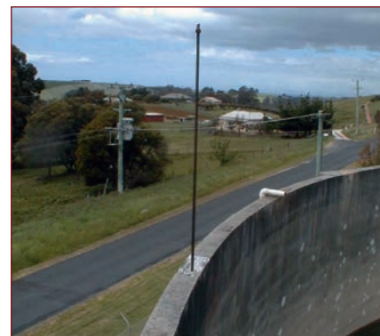
Figure 8. Failed vertical stressing bar from an approximately 3ML reservoir located on the North Coast of Tasmania.
