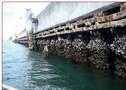
Figure 15. Above water view of sheet pile wall.
