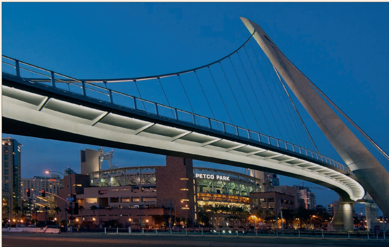
Opening in 2011, San Diego's Harbor Drive Pedestrian Bridge is one of the longest self-anchored pedestrian bridges in the world. Photo © Fred Kaplan.
