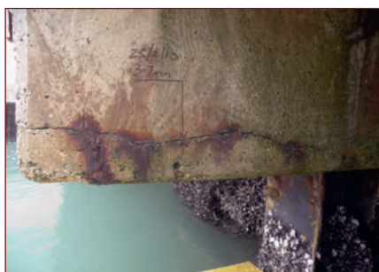
Figure 18. A crack at the edges / soffit of a dolphin structure.
