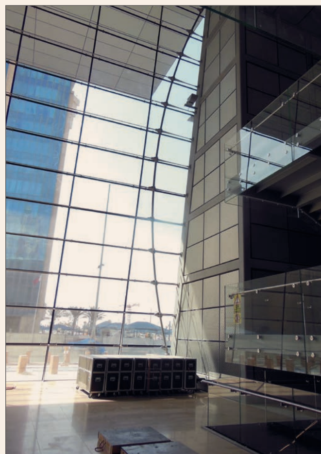
Located in Qatar, the Jahn-designed Doha Convention Center uses cable-net-supported glass walls to create a floating roof plane. Due to its structural properties and corrosion resistance, duplex stainless steel was specified for the façade. Photo courtesy Jahn.
