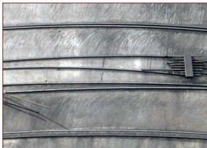
Figure 9. Failed post-tensioned cables on silos.
