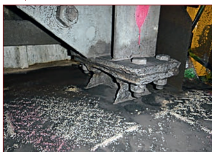
Figure 6. Column base plate has lost a large amount of section. Previous repair (coating only) inadequate.
