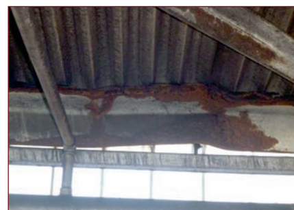
Figure 3. Failed top chord gantry compression member due to buckling at corroded area.
