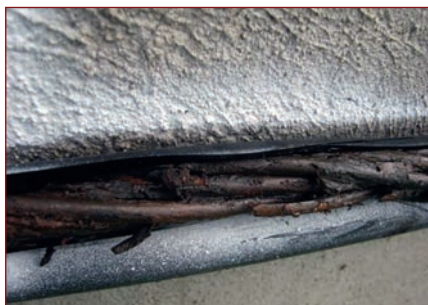
Figure 10. Corrosion to post-tensioned cables.
