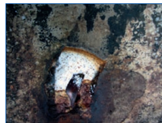
Figure 10. Example close-up of acidification induced deterioration to pile anode grout and concrete (typical).
