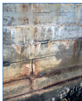
Figure 1. Example of deterioration/acidification of proprietary cementitious based backfill mortar within ribbon anode slots (typical).
