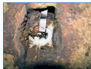
Figure 12. Example of loss of grout due to acidification and exposure of end of titanium current distributor (conductor bar) and end of anode (typical).
