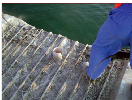
Figures 2 & 3: Impacting Method - Removal of deteriorated concrete by jack hammer.
