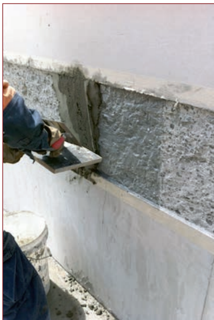
Figure 4: Concrete substrate is ready to receive repair materials after final surface cleaning.
