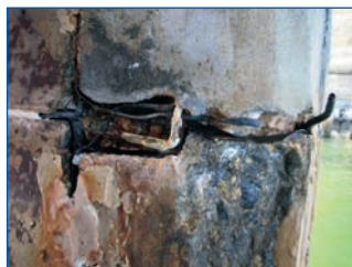
Figure 4. Example, another, of acidification and loss of backfill mortar to expose anode ribbon and anode connections (typical).
