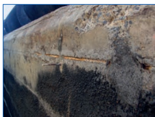
Figure 5. Example of local deterioration/acidification of proprietary cementitious based backfill mortar within ribbon anode slot (typical).
