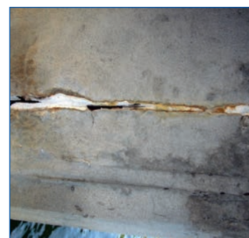
Figure 2. Example close-up of acidification and neutralisation of backfill mortar in ribbon anode slot (typical).
