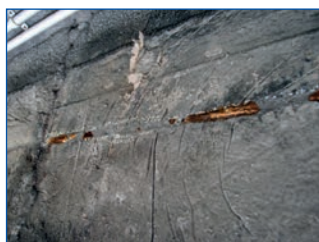
Figure 6. Example of local acidification and neutralisation of backfill mortar in ribbon anode slot (typical).
