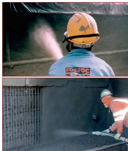
Figure 6: Sprayed repair mortar application .
