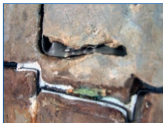
Figure 3. Example of acidification of backfill mortar to expose anode ribbon and anode electrical (positive) connection (typical).
