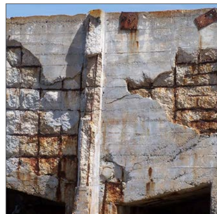
An abandoned building on Northern California's McAbee Beach shows the destructive power of corrosion on a steel-reinforced concrete structure. A new NIST evaluation method using terahertz waves can detect the early stages of corrosion on steel rebars directly through their concrete covering. Credit: With Permission by Per Loll, Denmark.
