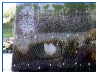
Figure 13. Example of electrocatalytically coated titanium mesh anode pinned to a bridge pier column concrete surface with plastic plugs and showing gap (~300mm) between anode zones as additional design means of managing current dumping (typical).
