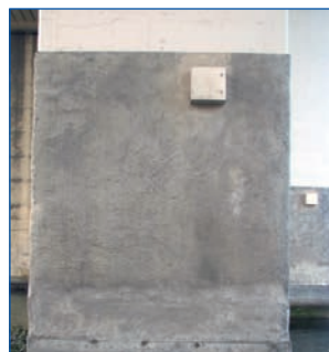
Figure 14. Example of cementitious overlay covering the titanium mesh anode to a bridge pier column in a marine environment (typical).
