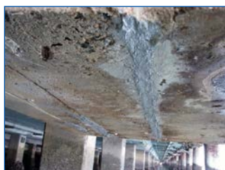
Figure 7. Example of localised "acidification" repairs undertaken by structure owner resources to wharf soffit element (see grey epoxy coating in photo) (typical).
