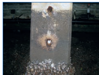
Figure 9. Example of acidification induced deterioration at pile anode locations (typical).
