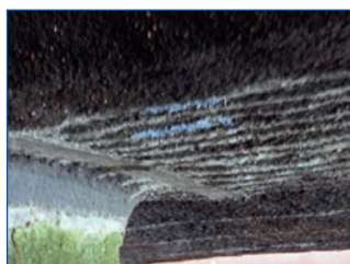
Figure 8. Example of localised "acidification" repairs to anode ribbon slots undertaken by structure owner resources (see grey epoxy coating in photo) (typical).
