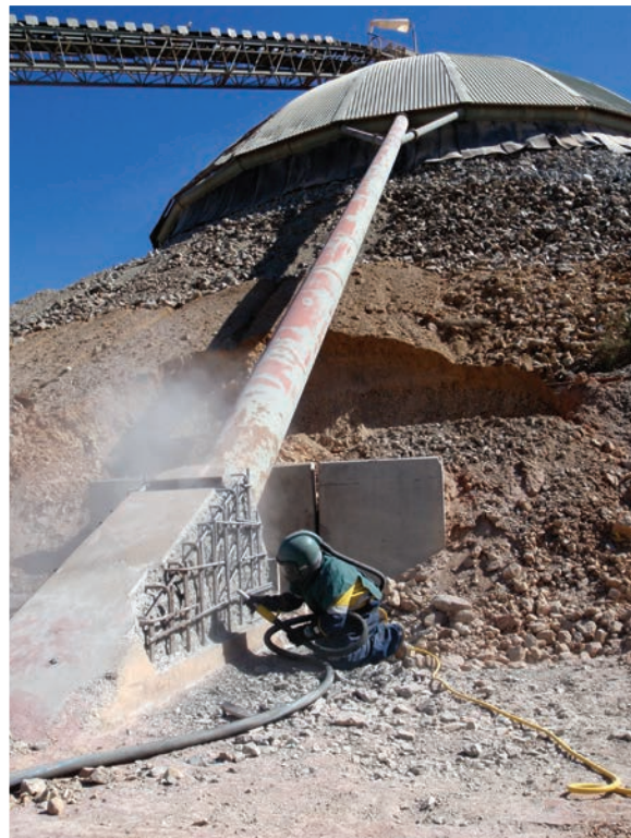
Front Cover Photo: Stock pile plinth concrete repairs at Kanowna Belle Gold Mine, 19 km north-east of Kalgoorlie. Photo courtesy Duratec Australia Pty Ltd.
