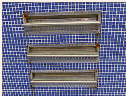
Figure 1: Stainless steel pool steps showing rust under cup nuts.
