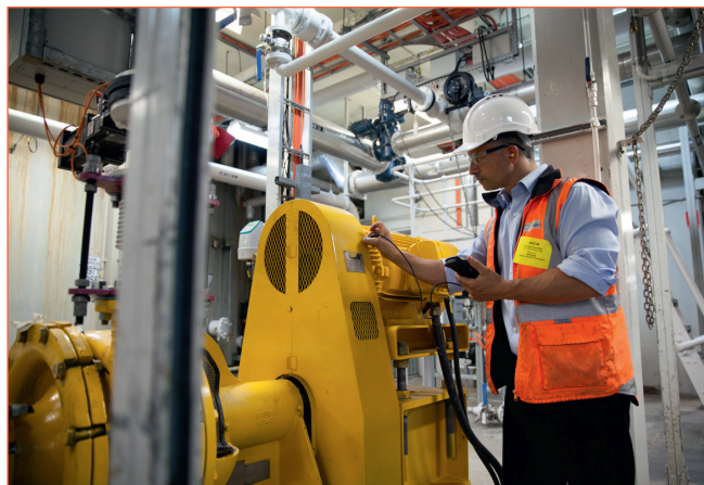
Coating film thickness inspections.
