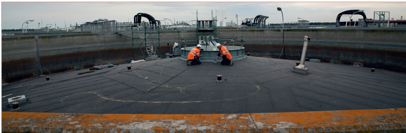
Installing reinforced geofabric liners.
