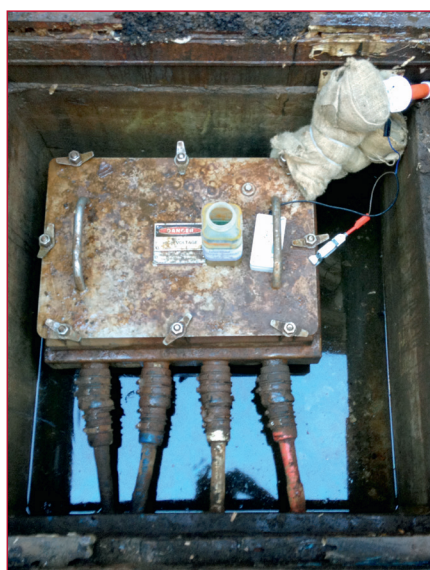
Figure 3 – 132kV Feeder cable earth link box.
