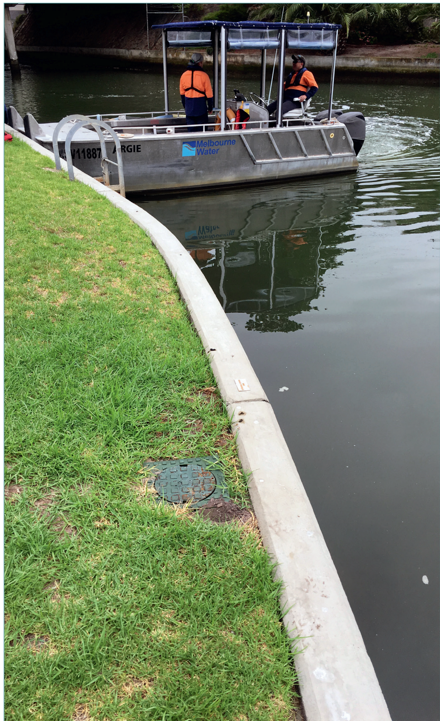
Figure 1. Electrolysis Test Point placed adjacent to wall and flush to ground level.
