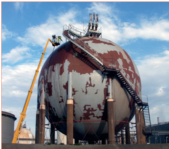
Lead paint removal.
