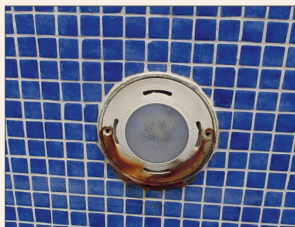
Figure 4: Severe rust staining on stainless steel housing of pool light.
