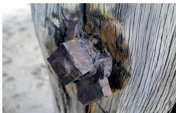
Above the waterline pier corrosion (VIC). Courtesy Robert Slater.
