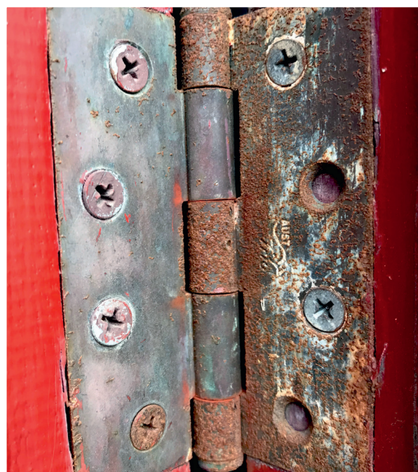
Brass plated Fe hinge on St Georges Cathedral (WA). April 2018. Courtesy I. MacLeod.
