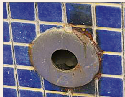
Figure 3: Corrosion on inner edge of pool water outlet vent.
