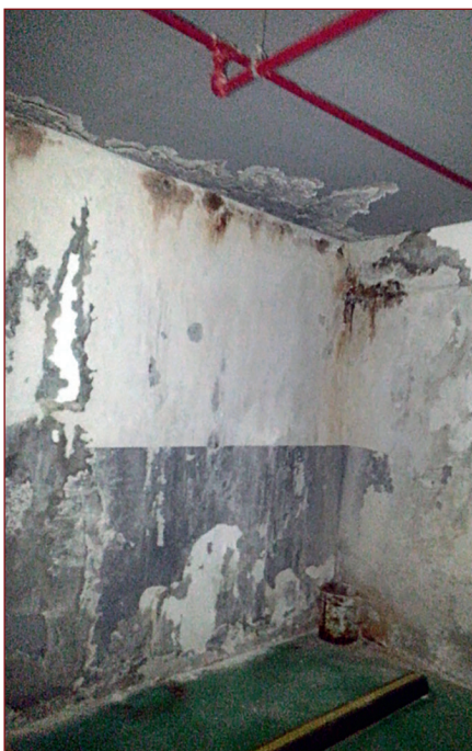
Leakage through retaining wall construction joint.
