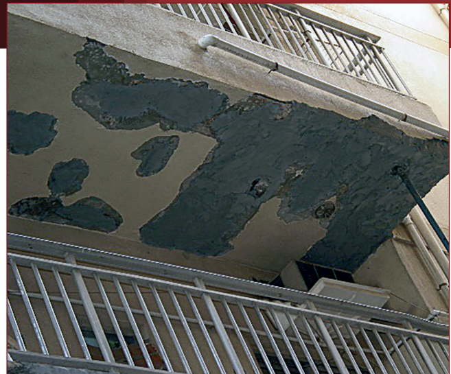
Damage from leakage in balconies.
