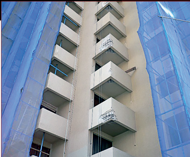
Balconies concrete spalling.
