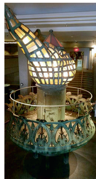
Original torch was replaced due to severe corrosion in 1986.
