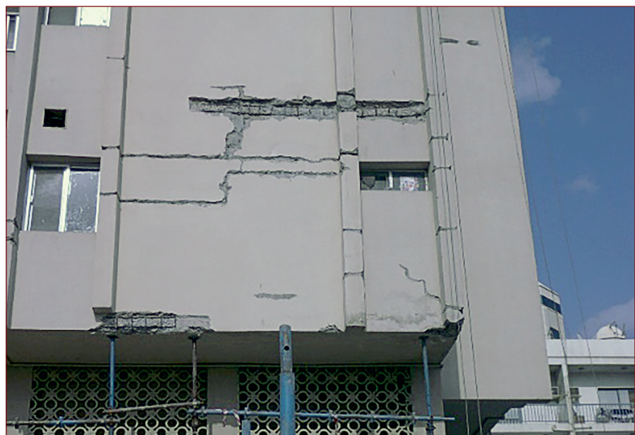
Water seepage from leaking bathroom to external building facade.
