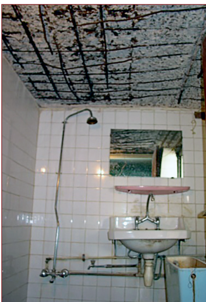
Bathroom ceiling corrosion problems in multi storey buildings.
