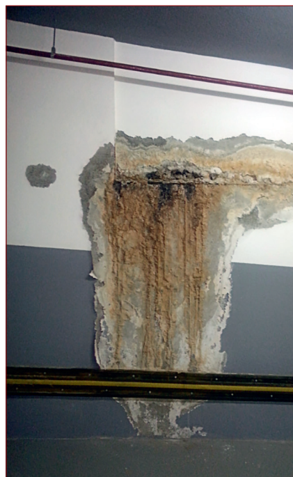
Basement leakage showing early signs of corrosion.
