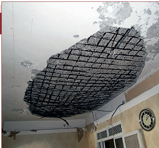
Roof leakage causes severe corrosion.
