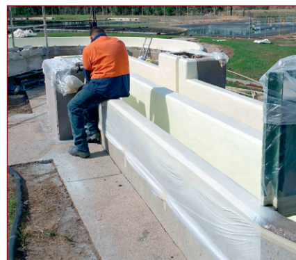
A grit channel and clarifier tank in the process of being coated.
