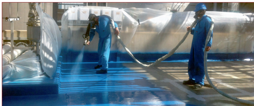
Technicians applying a coloured Pure Polyurea coating to hardstands at a chemical processing plant.
