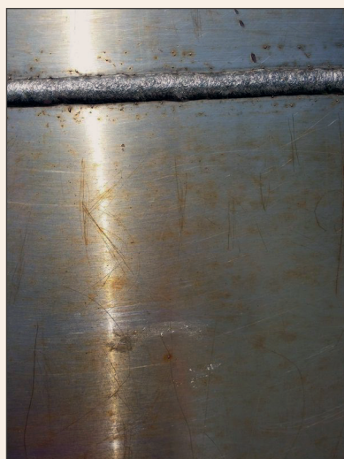
Figure 6. Superficial corrosion staining at the base caused by deicing salt exposure. [Photo taken by author in 2014].
