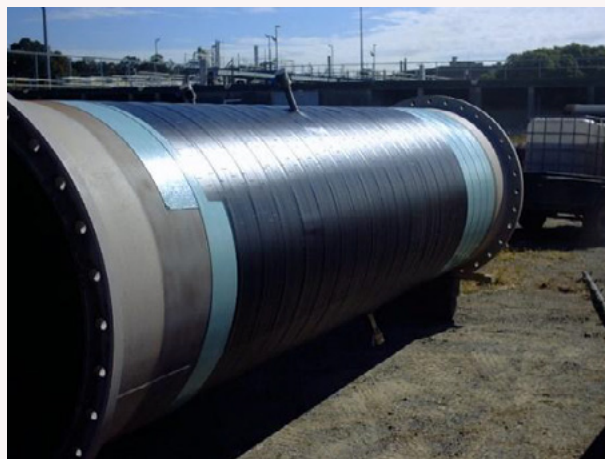
Figure 4: Application of the PVC outerwrap for UV protection of PIB system
