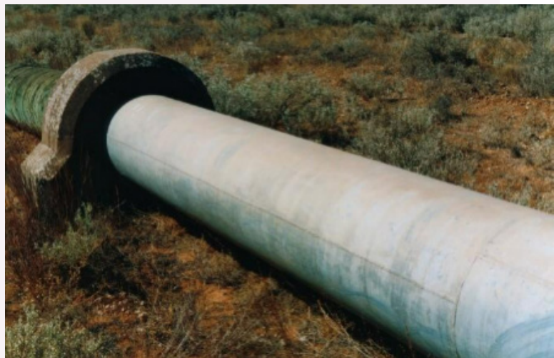
The Morgan-Whyalla pipeline was the first major structure coated with inorganic zinc silicate.
