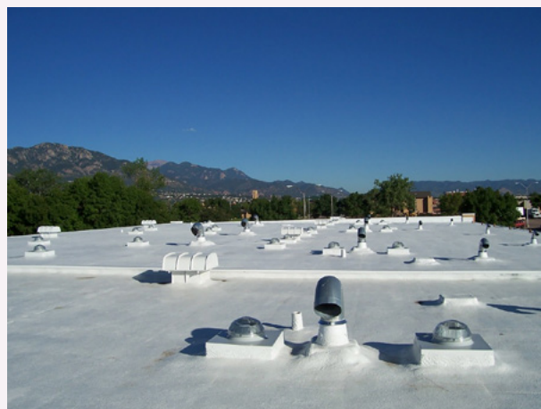
Figure 3. Recoated roof at Fort Carson
