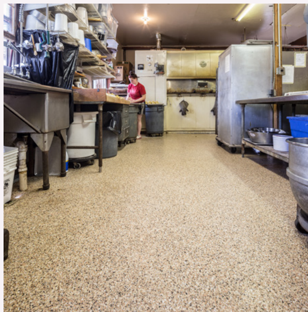
Figure 2. Finished polyaspartic floor
