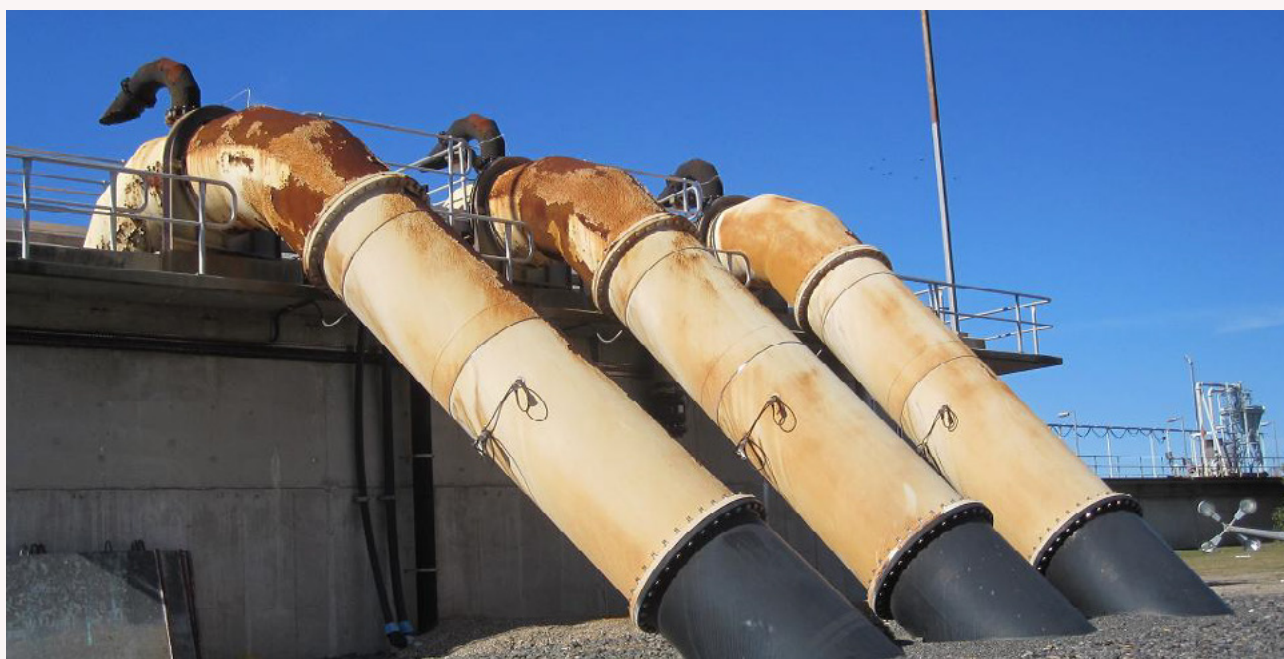
Figure 2 (below): Failure of traditional painted coating system on the steel pipe risers
