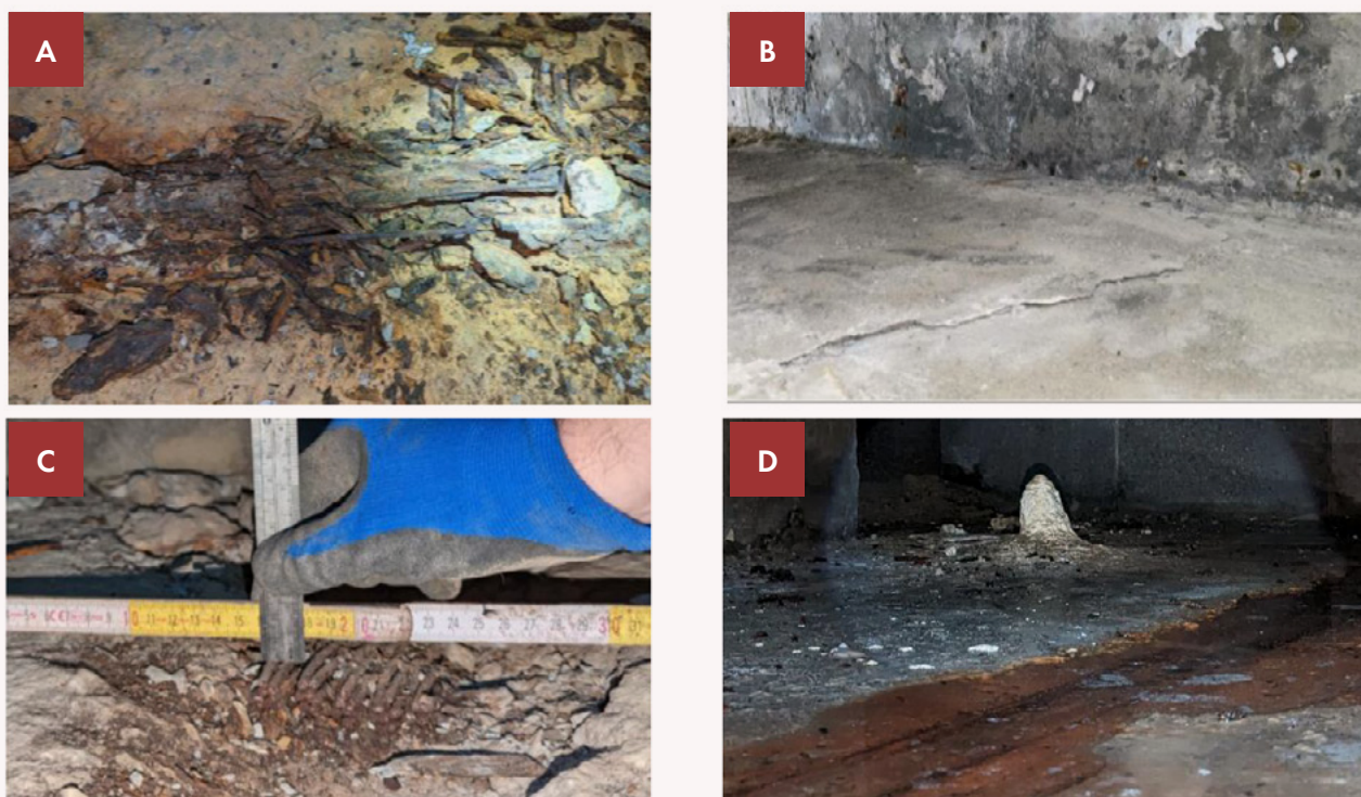
Figure 3. Deterioration observed within the services cavity. (a) Heavily corroded post-tensioning strand from the floor slab, (b) Efflorescence on pool walls and delaminated slab concrete due to strand corrosion (c) Low concrete cover (~10 mm) to corroded post-tensioning strands in slab in services cavity. Note that the duct has corroded away completely. (d) "Stalagmite" formed from salt and calcite deposits with delaminated concrete over low cover post-tensioning duct in the foreground.
