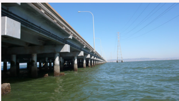
Figure 6. Coated pile caps on San Mateo Bridge
