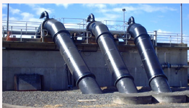
Figure 5: Completion of the PIB Coating system at the three main steel risers in 2011
