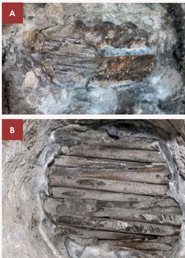
Figure 4. Water damage to strands and ducts. (a) Breakout of duct and strand within band beam, performed from above the beam in the area adjacent to the pool, (b) Breakout of duct and strand within band beam, performed from below the beam, showing strands in relatively good condition.
