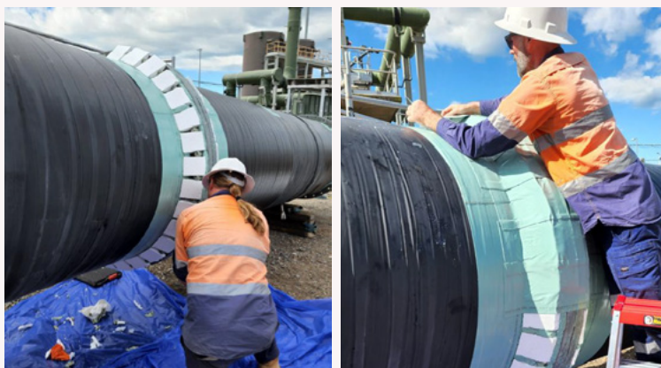
Figure 8: Upgrade of flange coating system with engineered foam wedges and re-application of PIB coating system.
