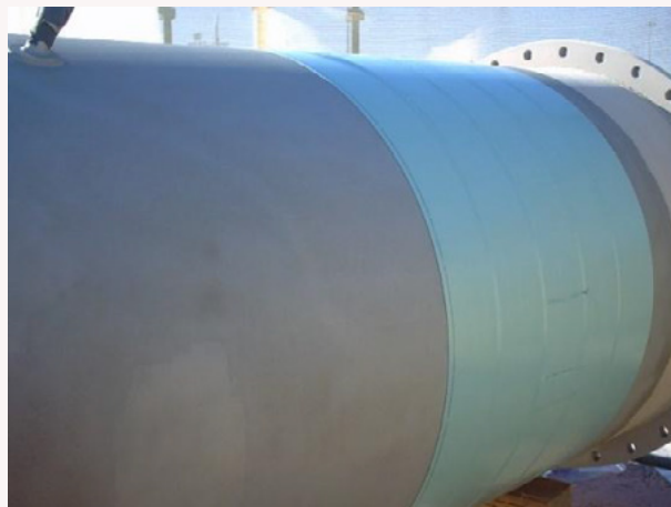
Figure 3: Application of the first layer of the PIB Wrappingband
