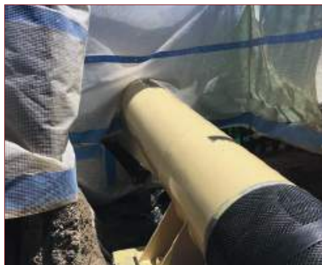
Recoated the above ground pipe section.
