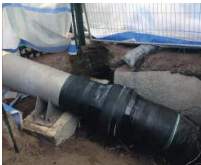
Pipe cleaned and recoated.
