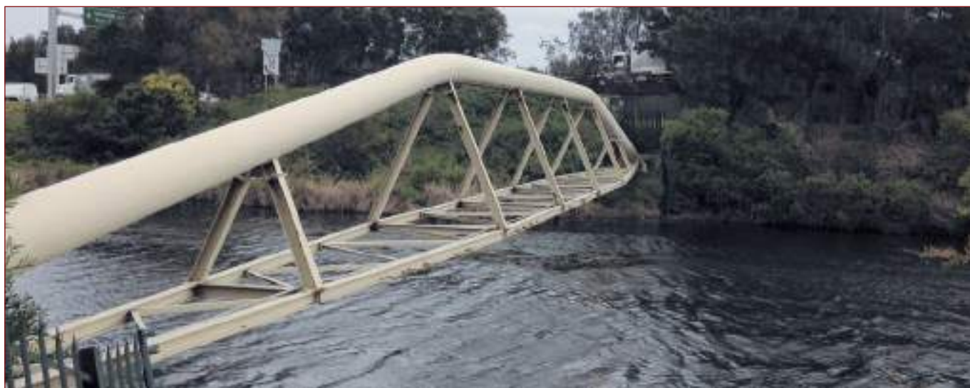
Pipe bridge crossing body of water.
