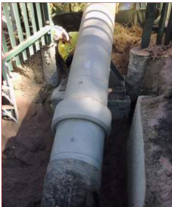
East End after Excavation.
